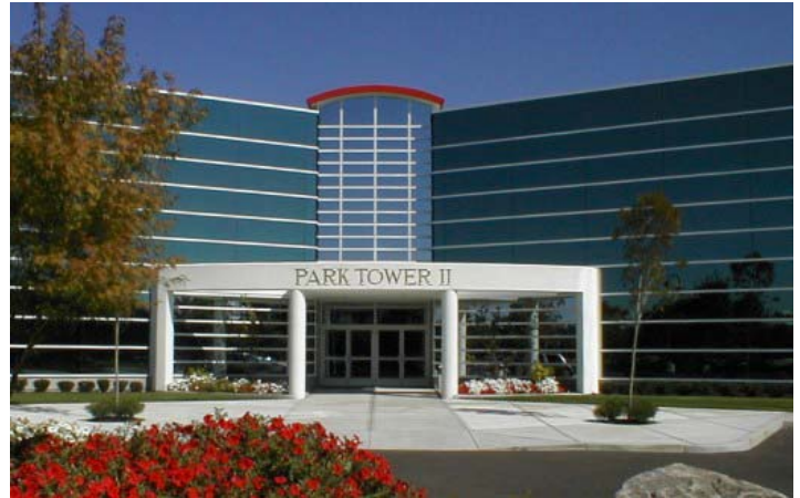
Jenkon's headquarters are located in the heart of the Pacific Northwest.
